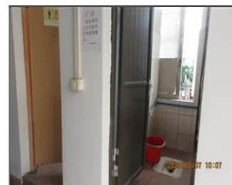
Photo of the sanitary facilities toilet.JPG
